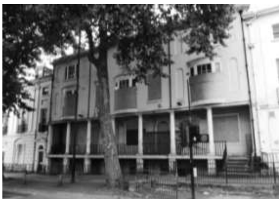
Pillar House, 19, 20 & 21 South Parade, built 1801
