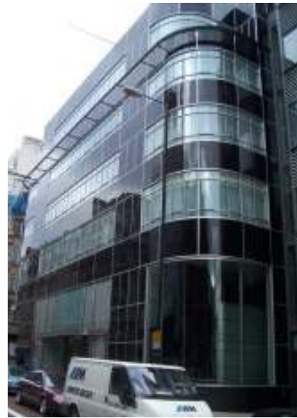
Former Daily Express, Fleet Street
