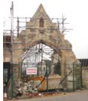
We felt that was still not good enough. The only real long term solution was to take down and rebuild the whole arch on a new foundation, given that it is currently supported by scaffolding. Losing a major architectural feature was not acceptable.
