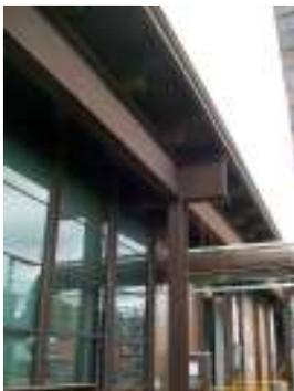
It was the first building in Britain to use Cor-ten, a steel which rusts to form a dark, purple-brown protective finish. Doncaster residents will never forget the “rusty car park” by North Bridge where the same steel had been fixed to enhance its concrete structure. Instead, it stained it rusty. But, when used correctly, the steel looks fine and never needs painting.
