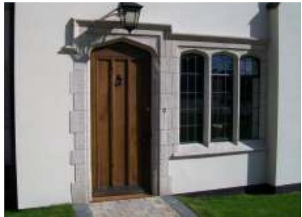
Handley Cross photographed in March 2014 with the development complete. The roofs have been re-laid in plain clay tiles, the render has been renewed, and the windows restored or replaced. The clay chimney pots are new.
