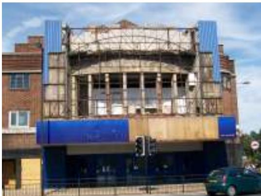
On Sunday 21 June 2009 the cladding was removed from the façade of the former Gaumont/Odeon cinema. There was damage to the curved high level balcony, which had been cut back to accommodate the flat metal framework for the cladding, and the restaurant glazing had disappeared (left).
