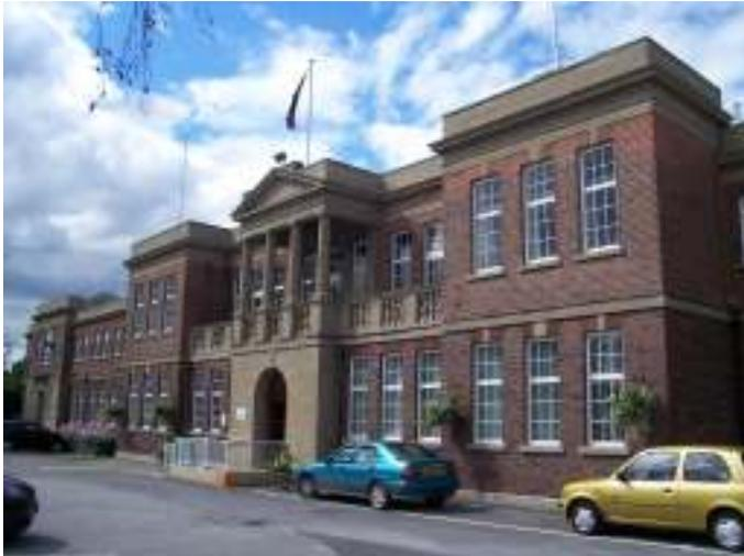
Perhaps the most significant renovation is the replacement of the 79 steel windows on the frontage with new ones in white powder-coated aluminium, in a matching Georgian style.
